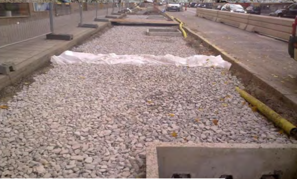
Layer for infiltration of rain water on top off the structural soil
