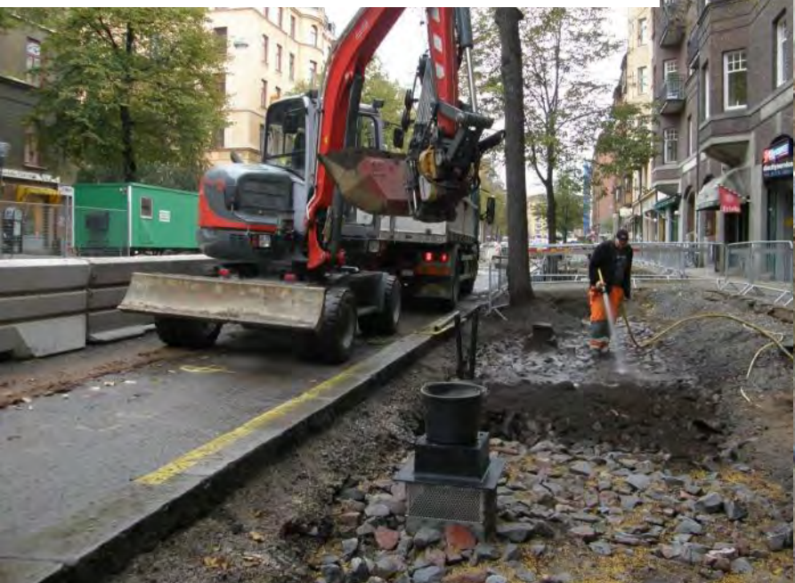
Flushing the soil into the structure
