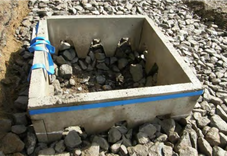
The stone shall fall into the box to get a stabel construction
