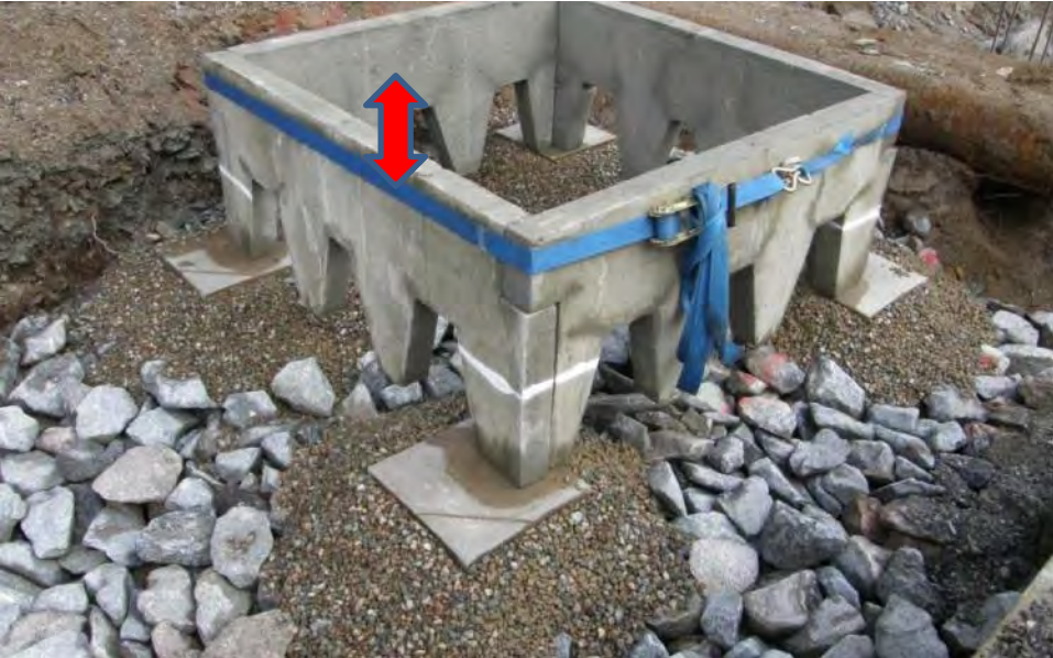
The stone shall fall into the box to get a stabel construction
